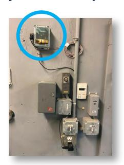
This wireless monitoring system allows you to remotely monitor temperature of a single device (TDX), or 2 devices simultaneously (TDX-Duo).
